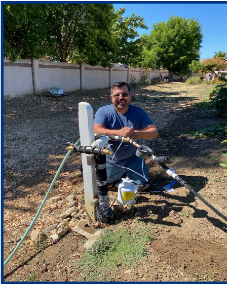
Some new plumbing parts donated by Nancy's Plumbing
